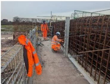
Image 1 North abutment reinforcement
