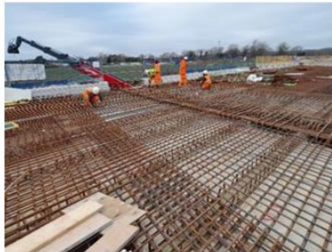
Image 2 Steel work progress
