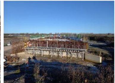
Image 3 View of viaduct facing North
